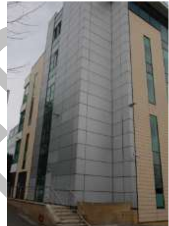
Figure 11: Ventilated cladding
