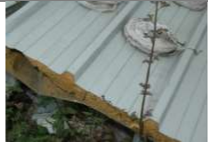
Figure 10: Non-ventilated cladding
