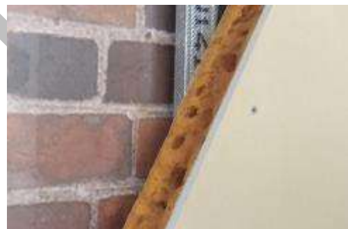
Figure 7: Combustible insulation
