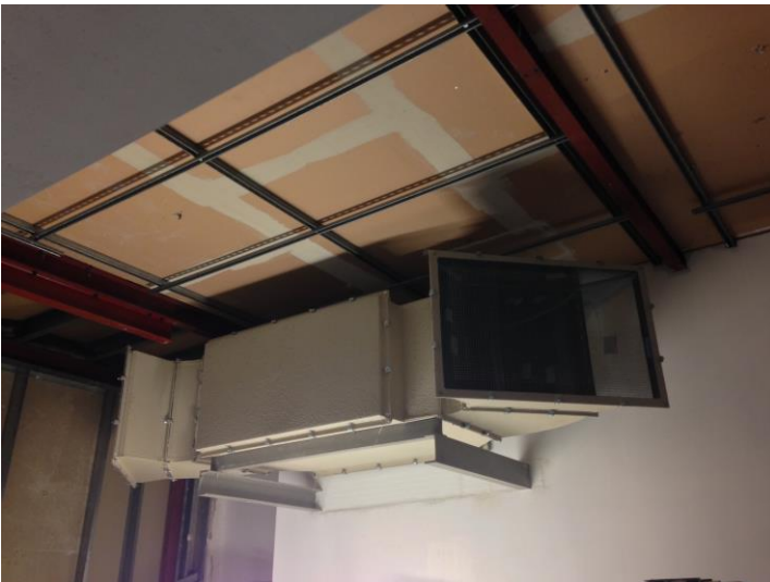
Figure 9: Smoke and heat exhaust ventilation system
