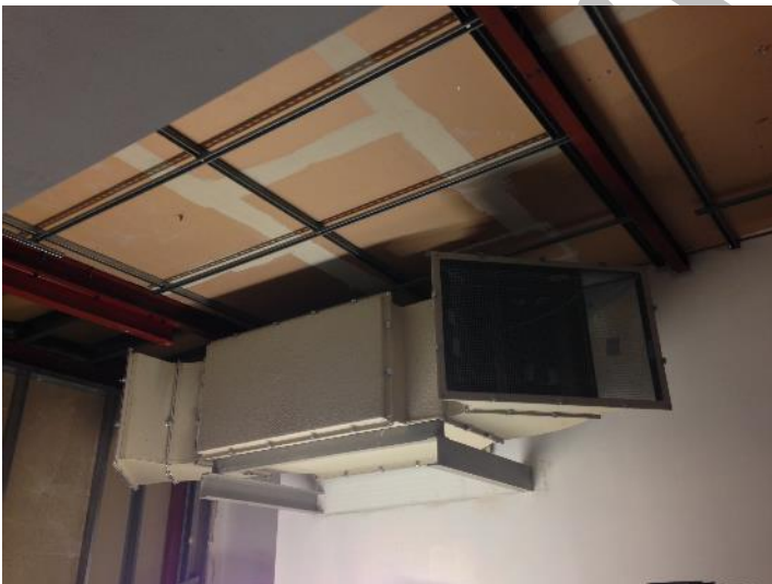
Figure 9: Smoke and heat exhaust ventilation system
