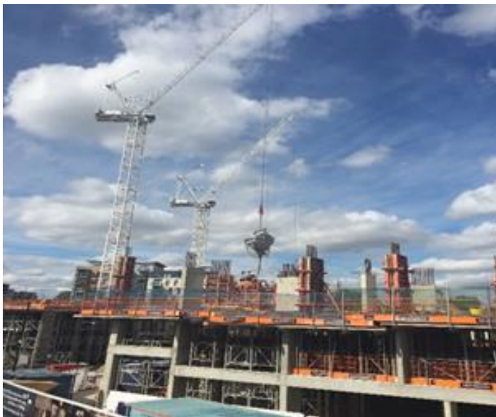
Figure 3: Large construction site – photograph courtesy of Brian Massie
