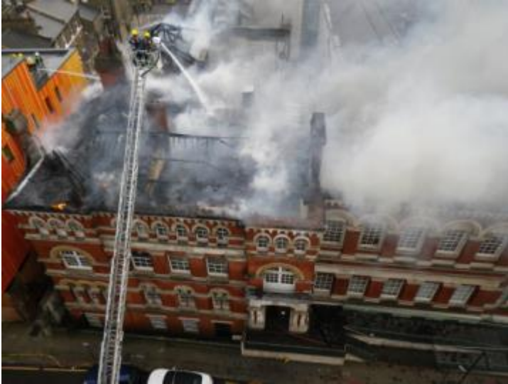
Figure 16: Fire in Walworth Town Hall, London, thought to have been started during building work to repair the roof – photograph courtesy of London Fire Brigade
