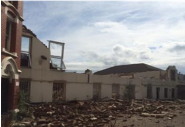
Figure 11: Demolition site showing rubble – photograph courtesy of Brian Massie
