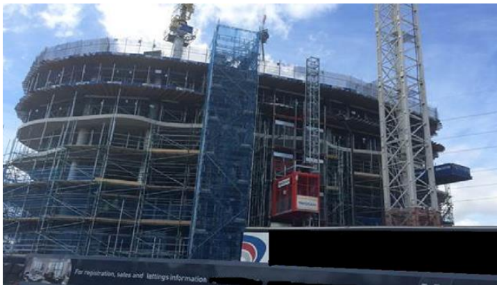
Figure 14: Scaffolding lift or 'hoist' – photograph courtesy of Brian Massie
