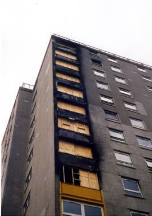
Figure 1: External firespread Source: Building Research Establishment
