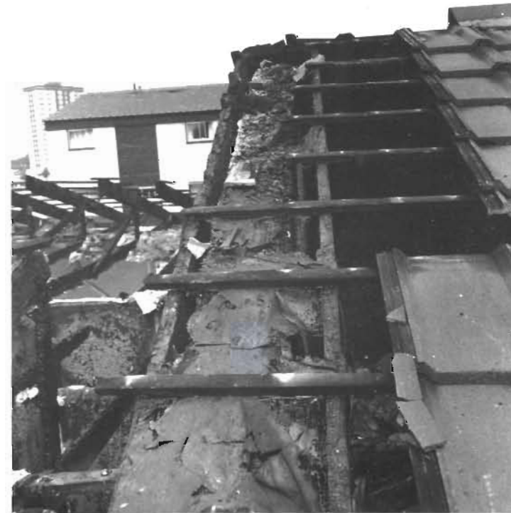
Plate 11. In this example of bad building construction the timbers have been set into the brickwork of the chimney flue which can be seen in the centre. Defective mortar allowed heat to reach the rafter which subsequently ignited. The resulting fire destroyed the top of the building.
