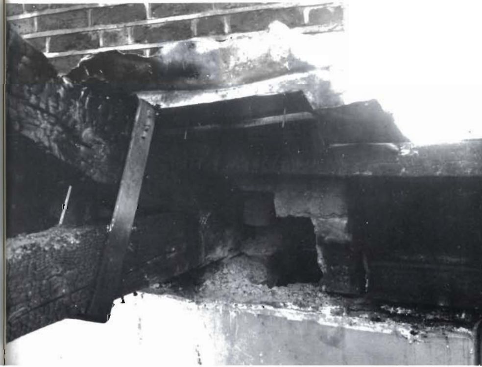
Plate 11. In this example of bad building construction the timbers have been set into the brickwork of the chimney flue which can be seen in the centre. Defective mortar allowed heat to reach the rafter which subsequently ignited. The resulting fire destroyed the top of the building.
