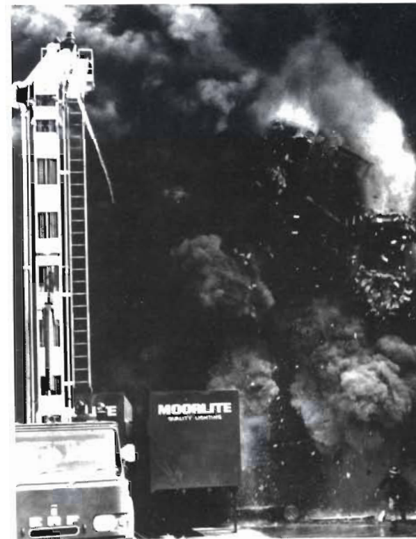
Plate 15 An almost explosive collapse of a warehouse wall which has, obviously, not given much warning. Photo Daily Express, Manchester
