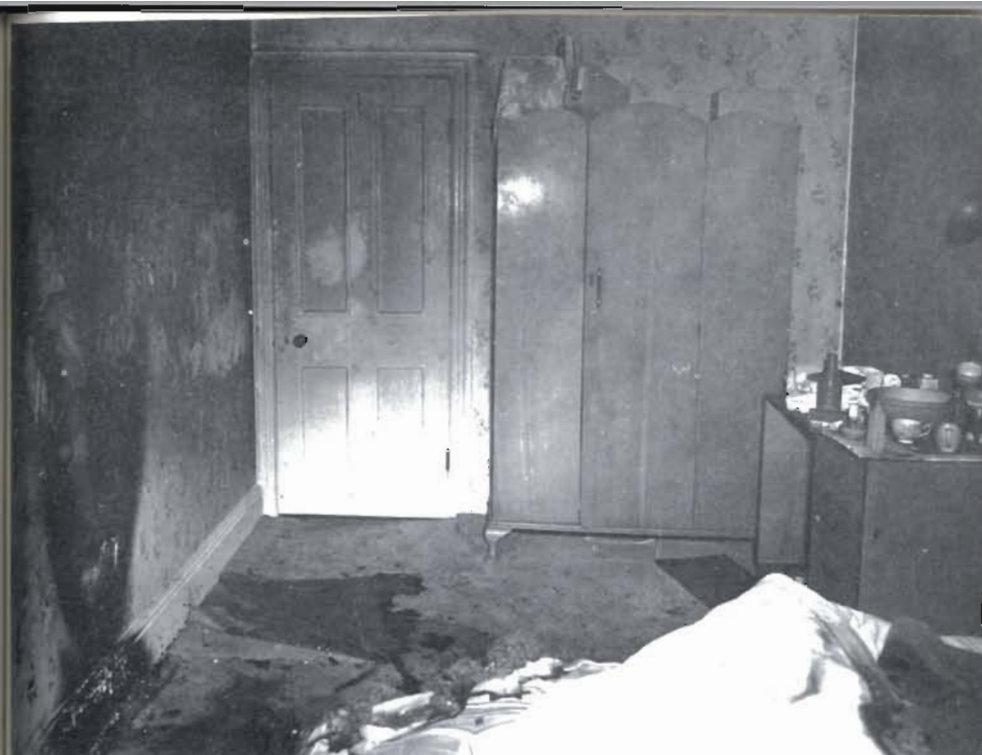
Plate 23 The pattern of damage strongly suggested that an oil heater had flared up without warning The presence of glass fragments implied a shattering of the drip-feed heater's glass container
