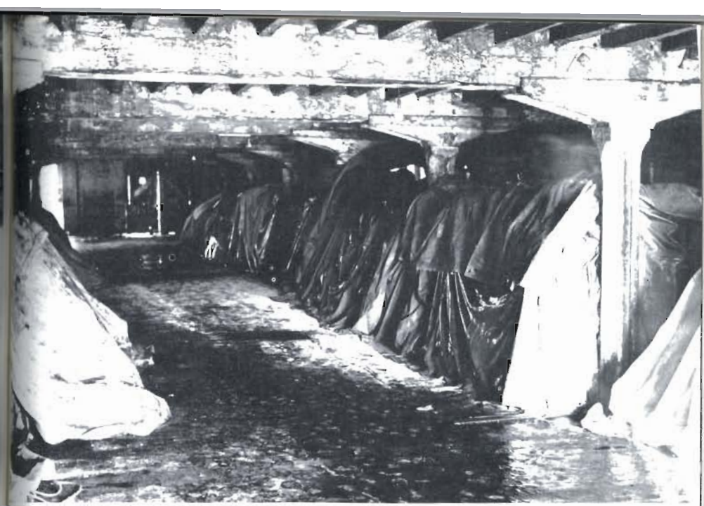
Plate 19 Goods in this warehouse are being protected by sheeting. The thorough covering and overlapping of sheets are particularly important Photo London Salvage Corps
