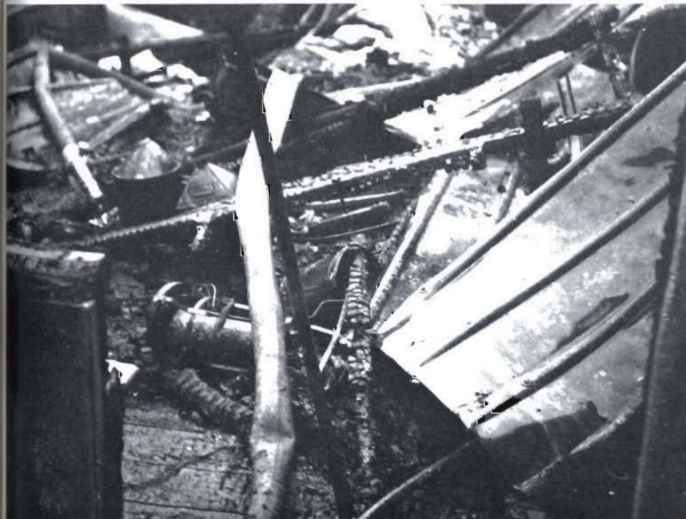
Plate 24 The presence of an oil heater, paraffin cans and a funnel at the site of this fatal fire suggested that the heater was being filled, but there was insufficient evidence for the coroner to record this
