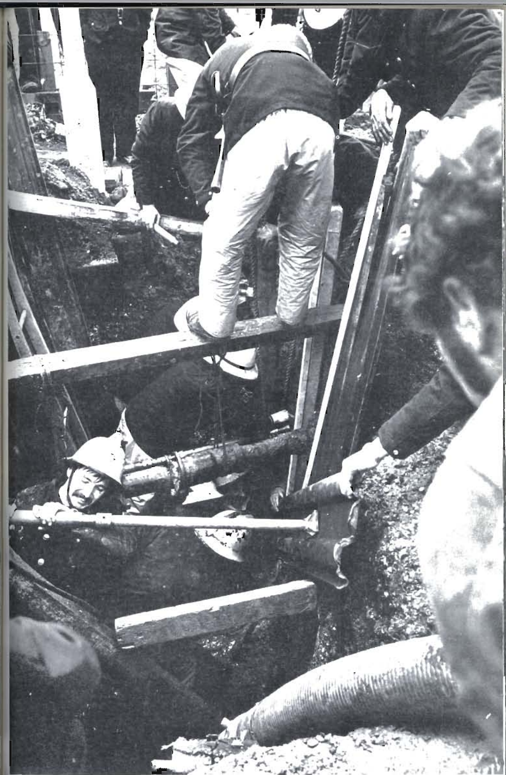
Plate 9 A special service rescue being carried out following the collapse of trench shuttering. Photo Birmingham Post and Mail
