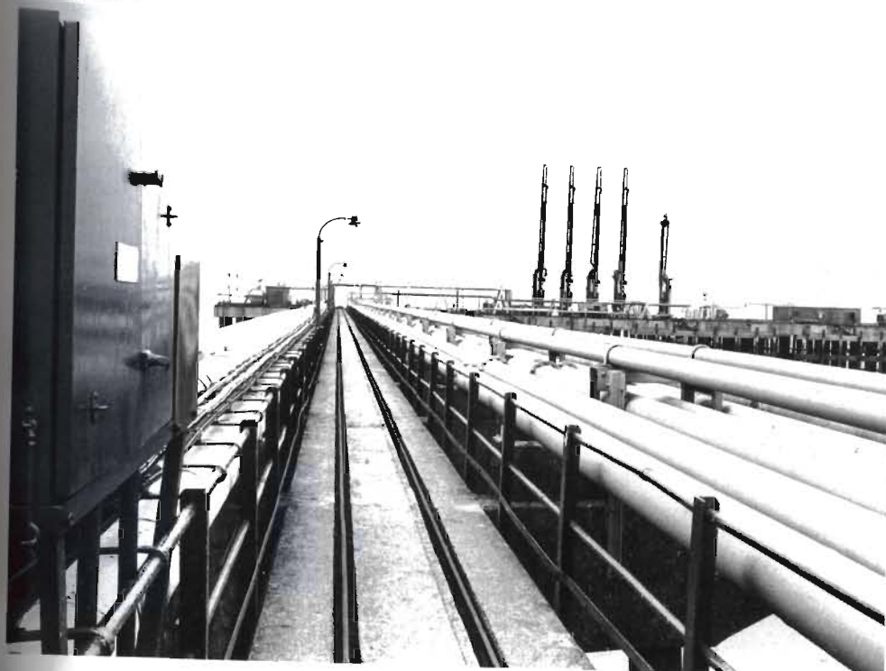
Plate S.10 An example of an offshore jetty leading to a marine refinery terminal. Compare with Plate S.11. Photo: Humberside Fire Brigade
