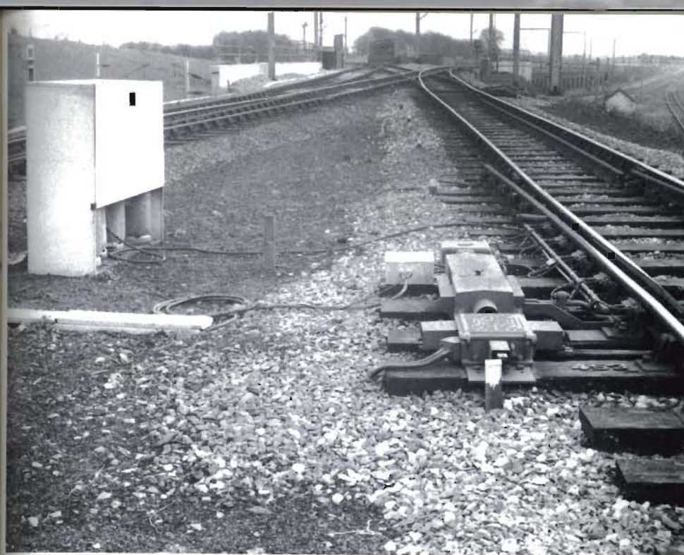
Plate R.1 Points, point operating mechanism, point heaters, rodding and LPG cylinders. Access to this particular place looks difficult.
