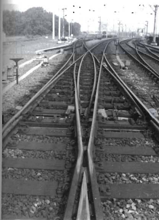
Plate R.1 Points, point operating mechanism, point heaters, rodding and LPG cylinders. Access to this particular place looks difficult.
