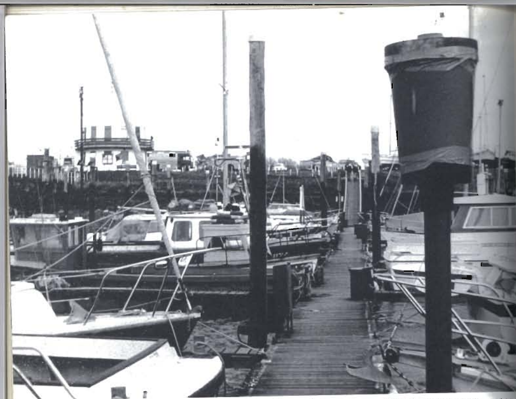
Plate S 11 This is the type of narrow, unlit, partially obstructed floating jetty which could be used for transporting equipment. Compare with Plate S 10. Photo: Essex Fire Brigade
