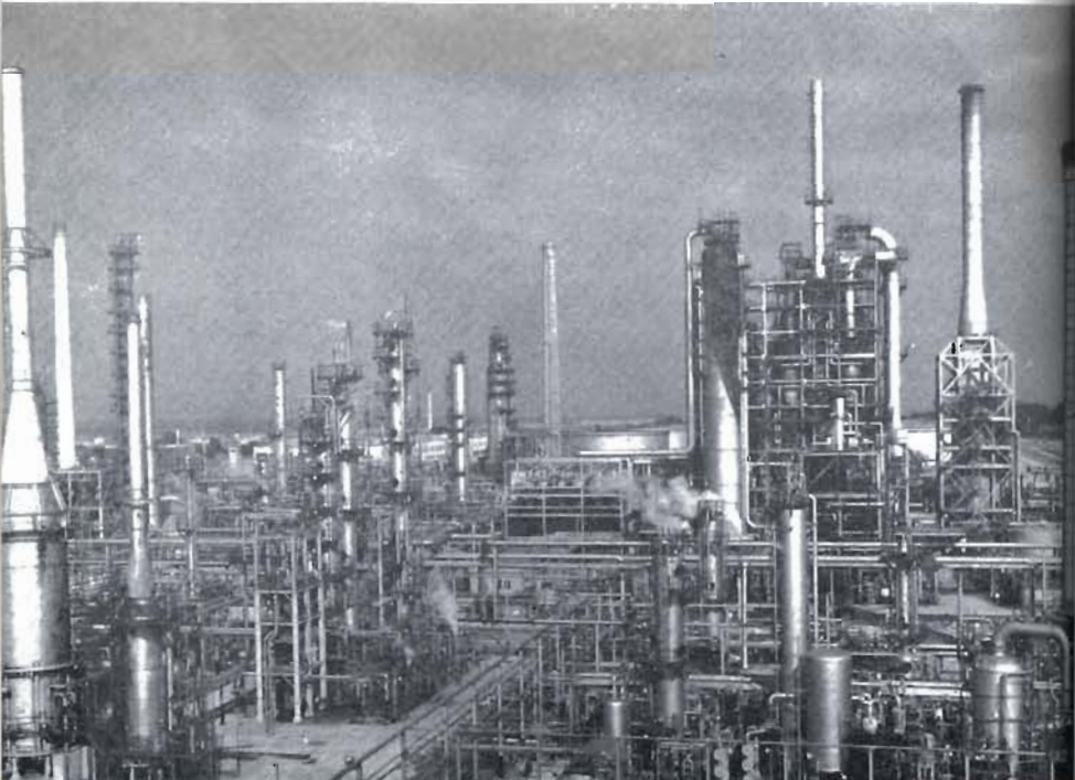
Plate 92. A typical example of the complicated mass of pipes and plant which is a feature of all oil refineries.
