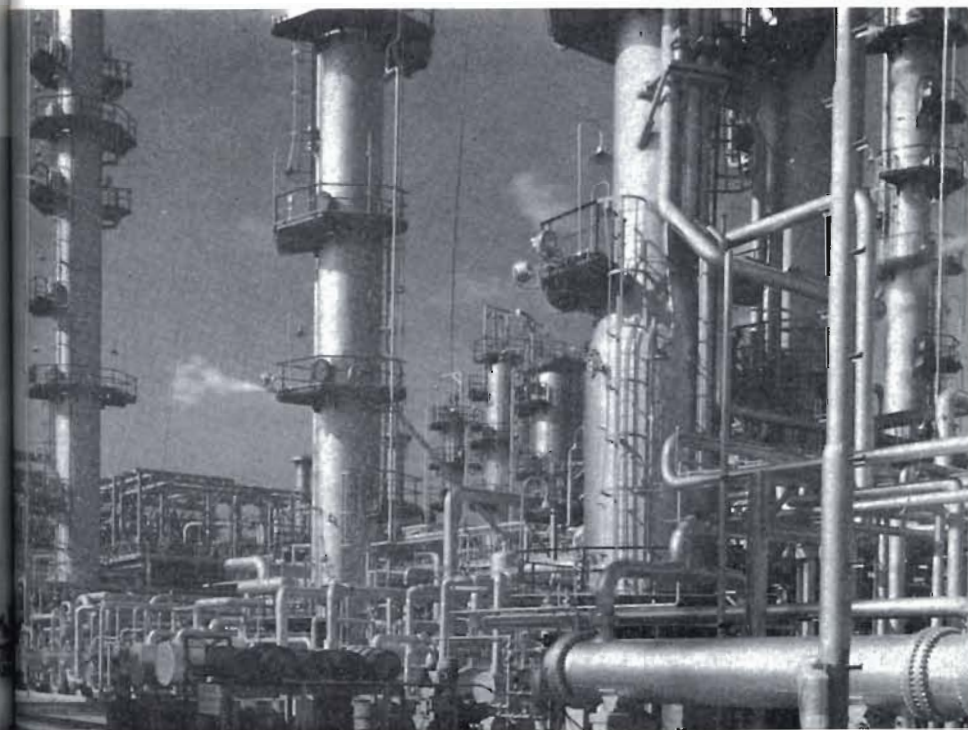
Plate 98. Chemicals are important products of an oil refinery. This is a general view of an ethylene recovery section of the chemical plant at Fawley. Much of this ethylene is supplied to the ICI plant at Severnside via a 78 miles (125 km) long pipeline.
