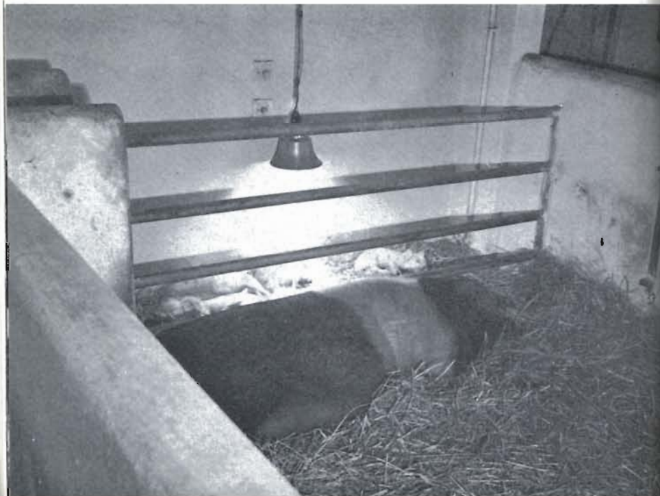
Plate 31. The type of heating and lighting used for rearing young piglets can be a source of danger from fire.
