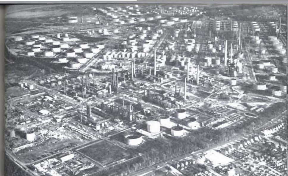
Plate 89. An aerial view of the Esso Refinery at Fawley, which occupies 1,250 acres (506 hectares).
