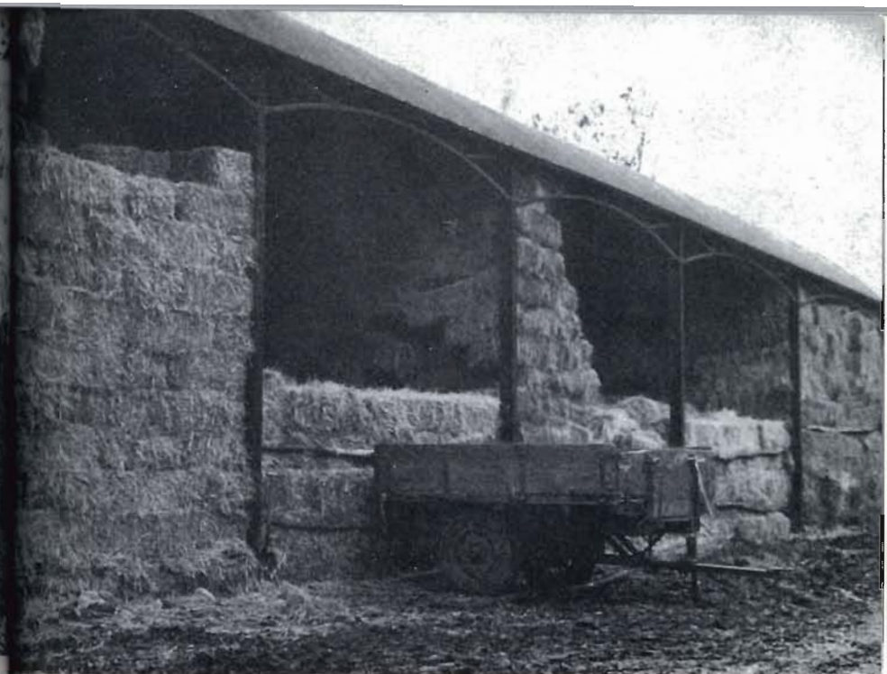
Plate 20. A typical 5-bay Dutch barn used for storing baled hay or straw.
