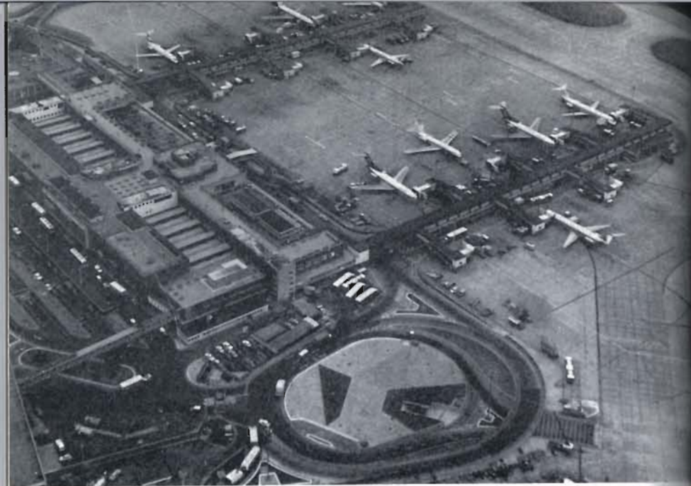
Plate 66. The passenger walkways (also known as fingers) and nose loaders at one of the aircraft aprons at Heathrow Airport.
