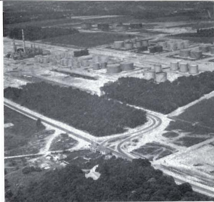
Plate 93. An example of the BP integrated refinery at Vernon, near Paris. Particular attention has been paid to landscaping of the site.
