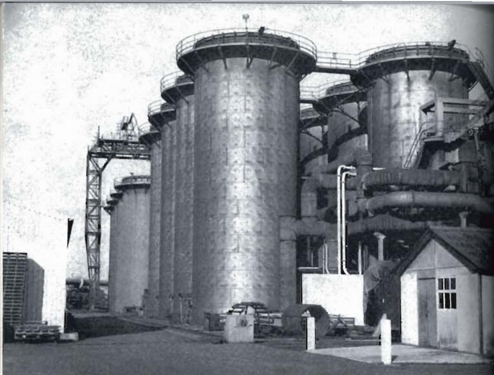
Plate 35. Tower purifiers which may be found at older gasworks.
