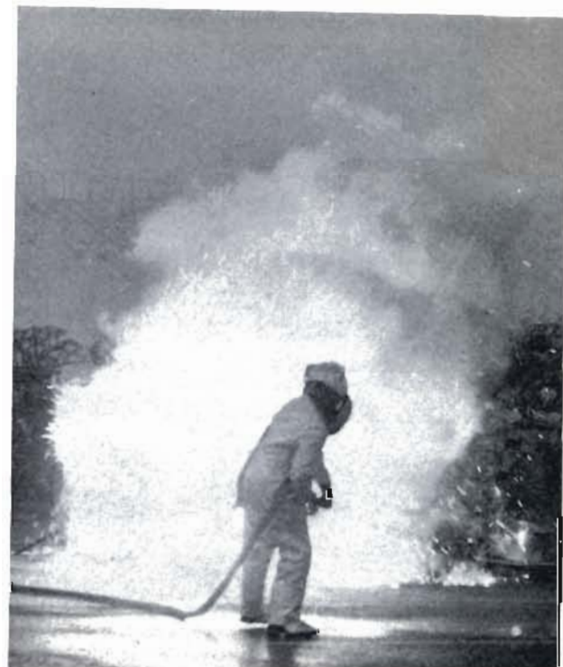
Plate 69. A demonstration showing the effect of water on burning magnesium.
