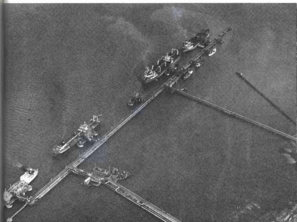
Plate 90. The Esso marine terminal at Fawley; this is 4,200 ft. (1,280 m) long and has five berths for ocean-going tankers. The berth at the top of the picture can accept partly laden vessels up to 300,000 tons (305 000 tonnes).
