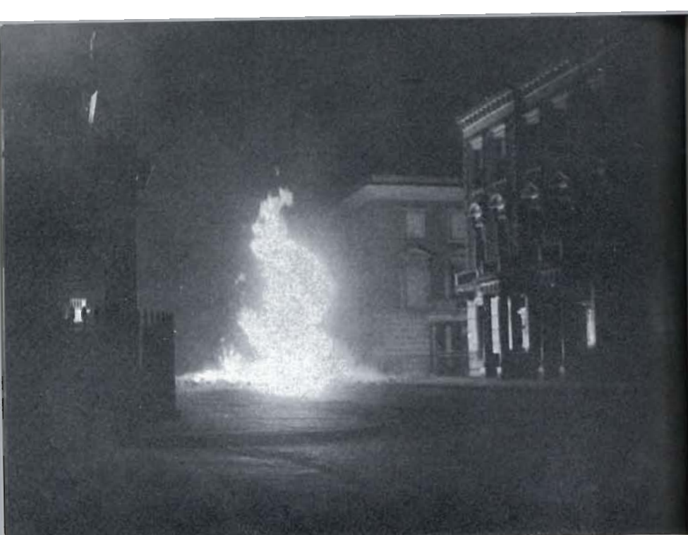
Plate 43. Gas burning from a damaged gas main.
