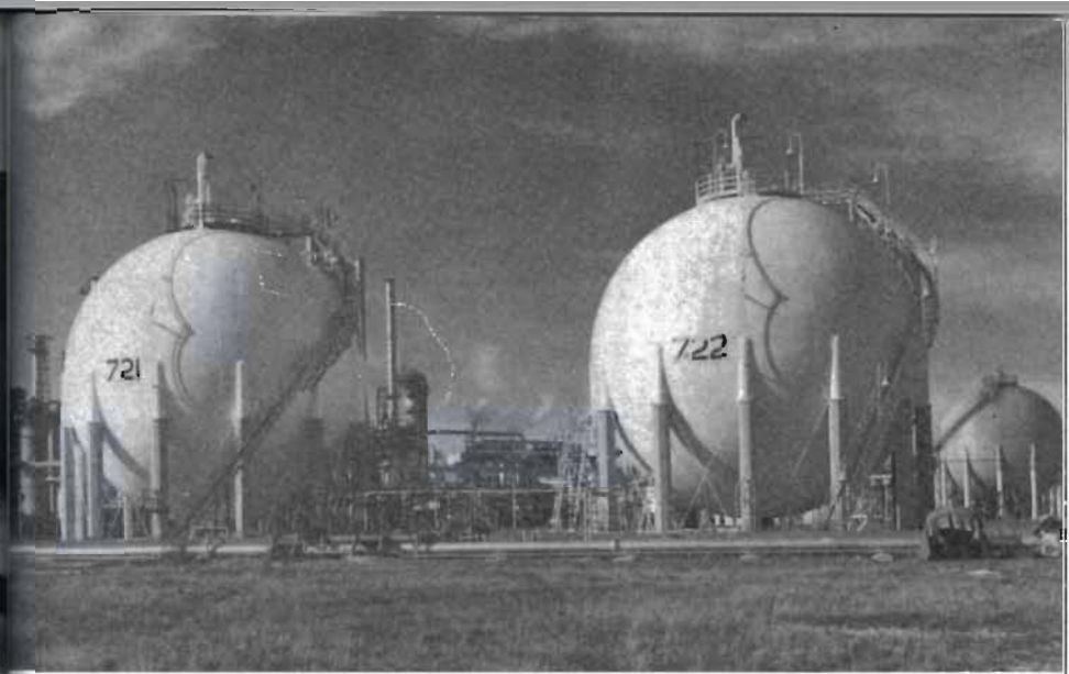
Plate 101. Spheres used for the storage of liquid butane gas under pressure. These have a capacity of about 1,000 tons (1 016 tonnes) each.
