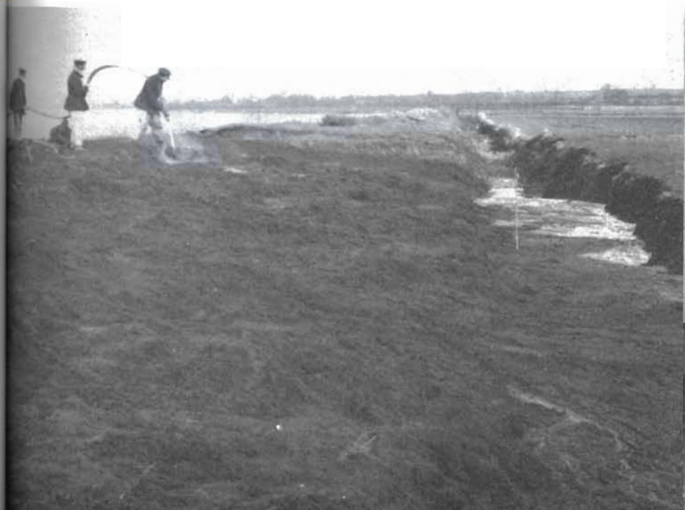
Plate 17. The result of fire-fighting operations in the peat-land fire shown in Plate 16. Loose peat ash is being washed into the dyke.
