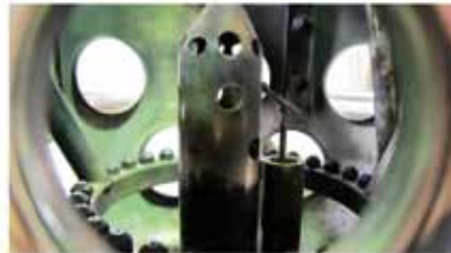
Pilot light and Burner Ring
