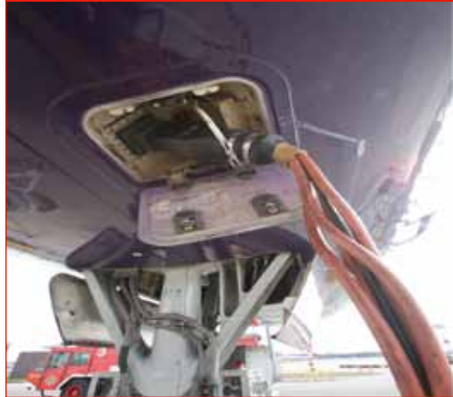
Picture 15: Fixed ground auxiliary power unit connected to the electrical intake of a civil aircraft
