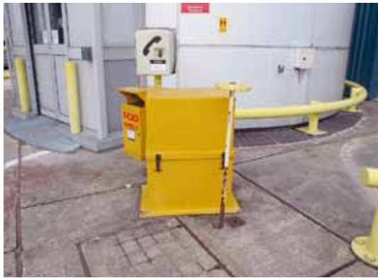
Picture 24 and 25: Pillar hydrant and control valves with insulated boxes
