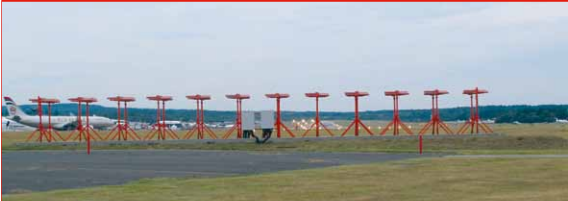
Picture 2: Instrument Landing System (ILS) Farnborough Airport
