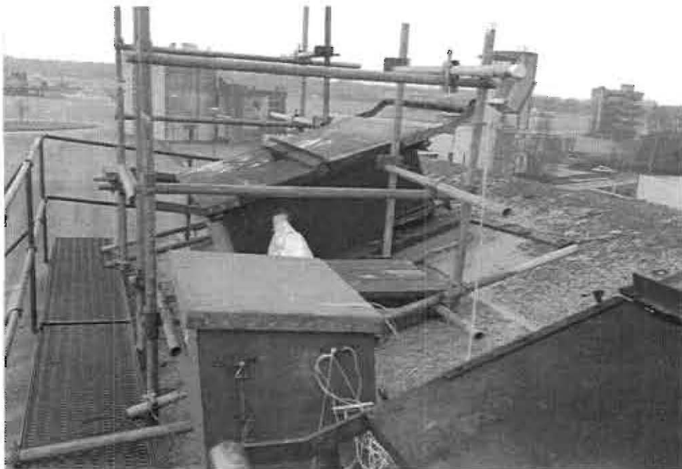
Figure 6 : North vent showing scaffolding and protective box for instrumentation
