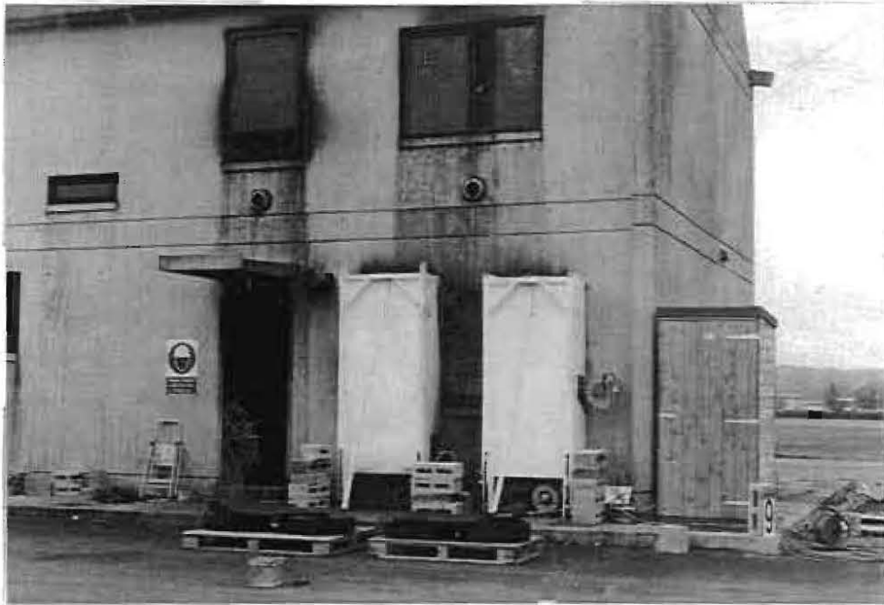
Figure 11 The Smoke Retaining Boxes in Position at Window Openings
