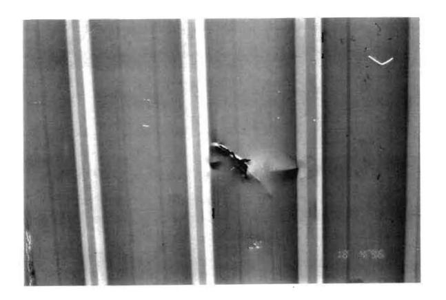
Exterior wall of building showing puncture (from fork lift truck).
