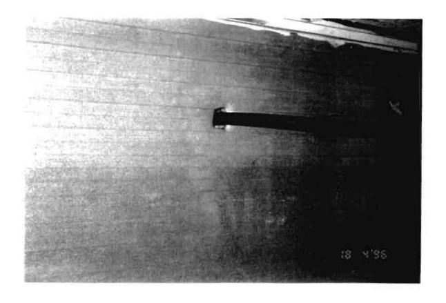
Penetration of services through ceiling panels Note ice build up on pipes.
