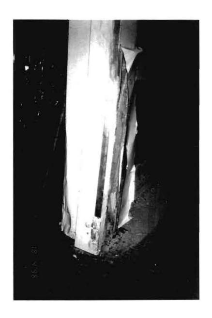
Typical impact damage to door frame base (from fork lift truck)
