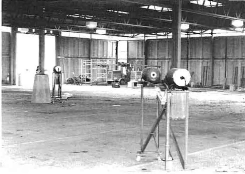
Figure 5. The 'green' garage; internal view, with door open at left.
