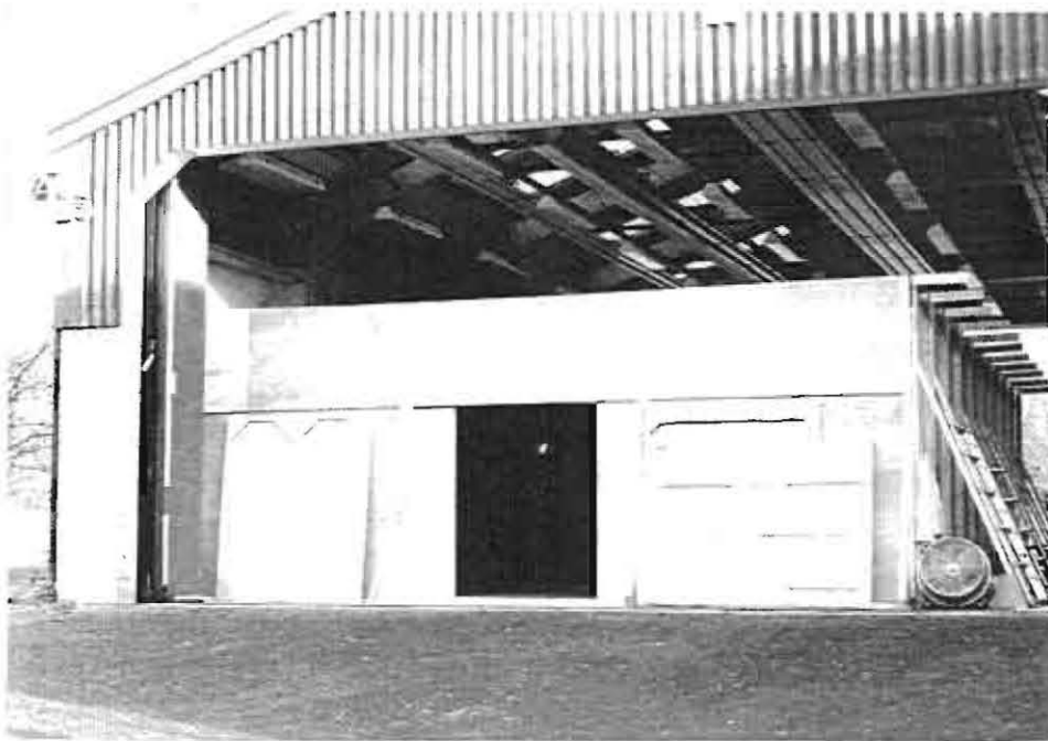
Figure 14. Temporary building – 7.0 metres wide with 1.52 metre (5'-0") wide central doorway.
