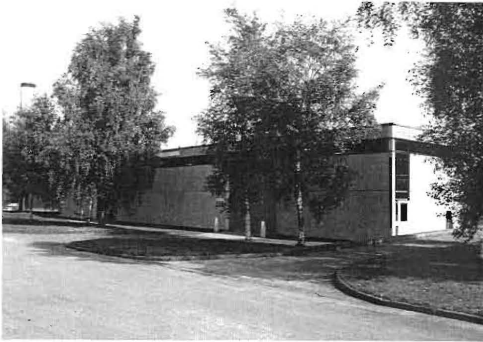
Figure 3. The 'green' garage: general view.
