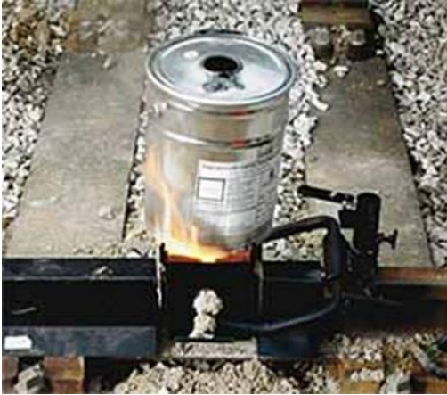
Figure 10: Example of track welding powder on a track Source: Open source
